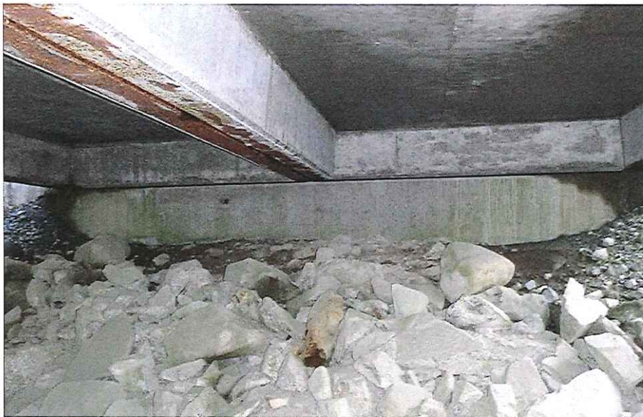
CK2097 Abutment Right Bank
