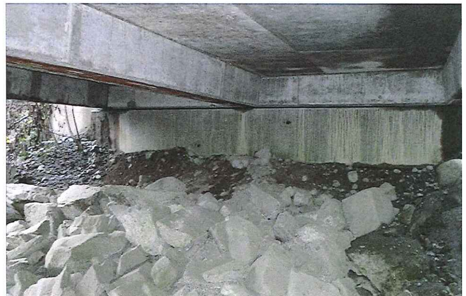
CK2097 Abutment Left Bank
