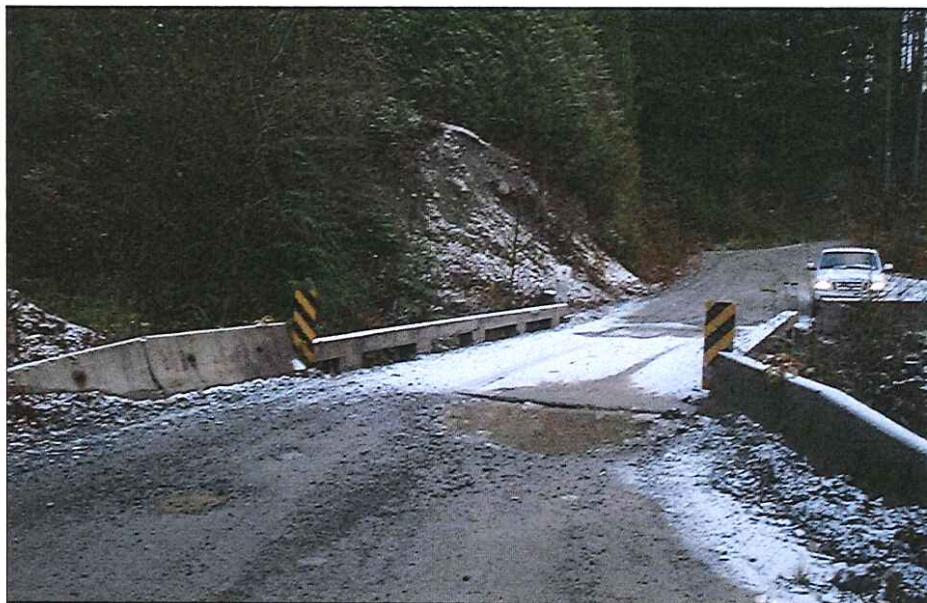
CK2097 Approach Right Bank
