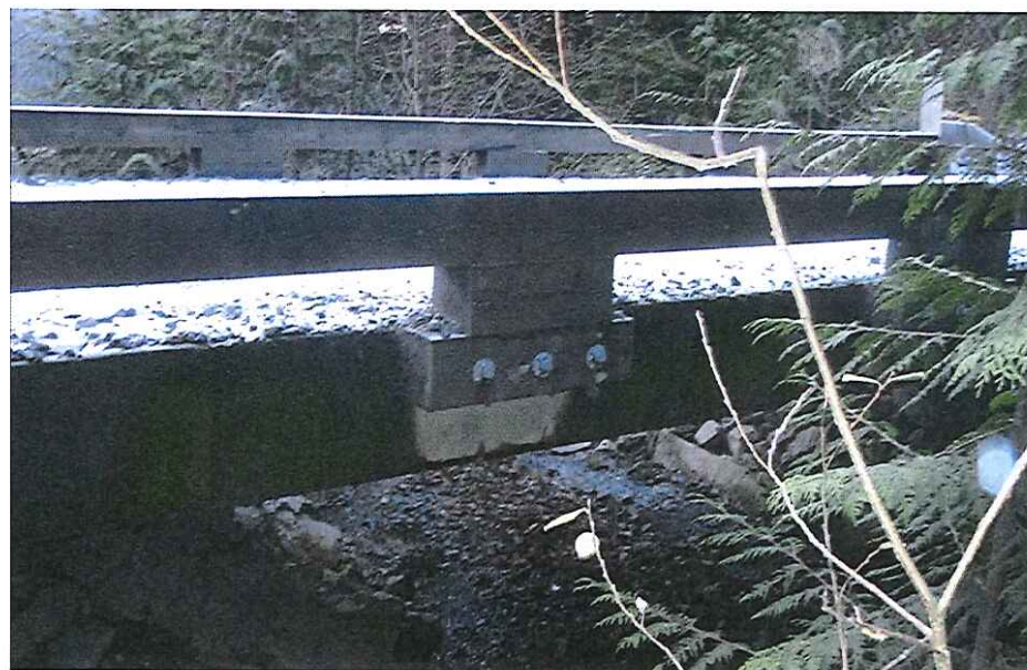
CK2097 Crossing Upstream
